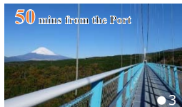
50 mins from the Port ⑬ Mishima Skywalk Parking: 400 cars Japan's longest pedestrian suspension bridge.
