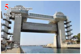
⑤ Large Flood Gate and Observation Deck, View-O
