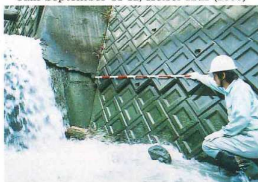
Crack appeared on the bank protection at the toe portions of the landslide.
