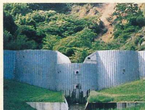
Nakayamasawa in Kawazu River drainage (Yugano, Kawazu Town). The steel made cell dam first constructed in Shizuoka Prefecture, H: 12m, L: 49.5m (Heisei 3th (1991))
