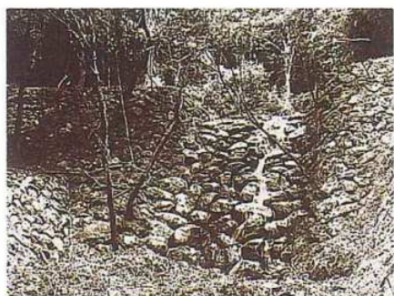
Konnosawa torrent in Ohi River drainage (Okusa, Shimada City). Check dam covered with stones constructed in Taisho 2th (1913)
