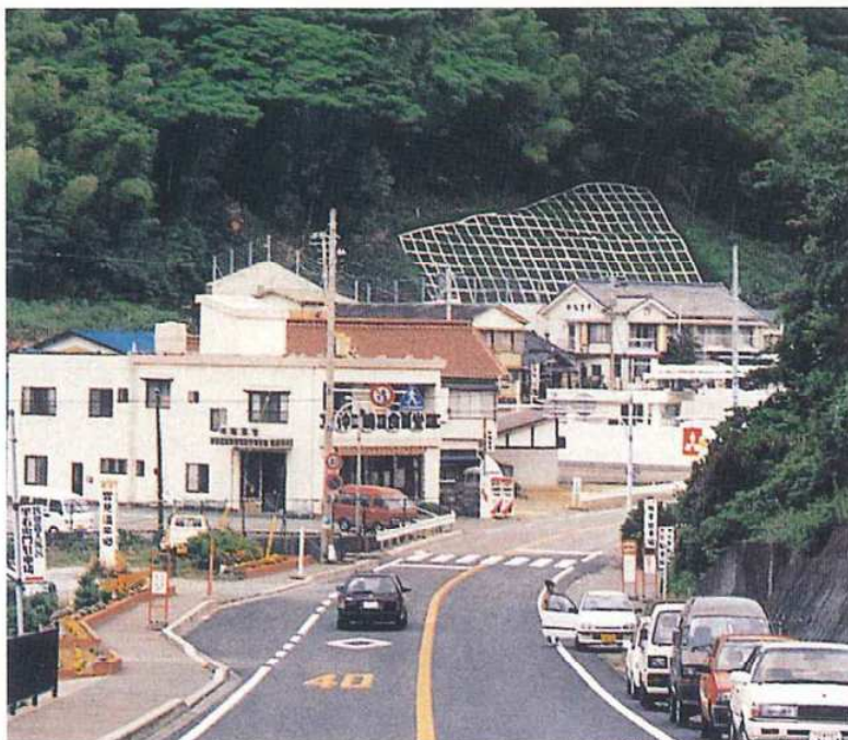
Steep slope protection facilities for protecting houses and emergency transportation roads. Steep slope at Kumomiukenoyama (Kumomi, Matsuzaki Town)
