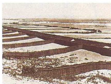
The right bank at the mouth of Ohta River (Fukude, Fukude Town, Iwata County). Flying sand prevention works at the seaside of the river mouth in Showa 14th (1939)
