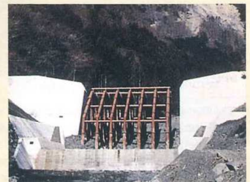
Skamoto River (Kuchisakamoto, Shizuoka City) Open-type steel-pipe gridded Sabo dam (Heisei 12th (2000))
