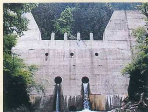
Izunuma River in Tenryu River drainage (Urakawa, Sakuma Town) Steel slit dam, first constructed in Shizuoka Prefecture (Showa 57th (1982))
