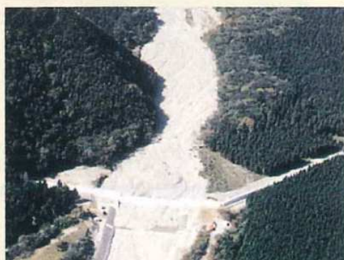
Fumotogawa in Fuji River (Fumoto, Fujinomiya City). The longest check dam in Shizuoka Prefecture, H: 6m, L: 262m (Heisei 2th (1990))
