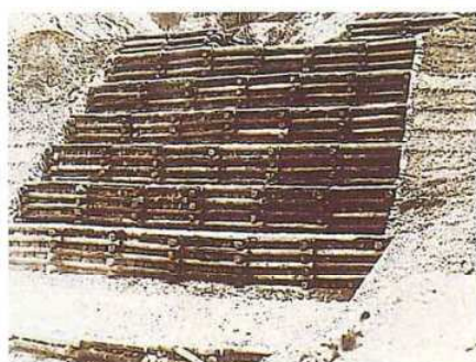
Kiriyamasawa torrent in Ohi River drainage (Ieyama, Kawane Town). Kiriyama No. 2 check dam made with wood in Showa 9th (1934)
