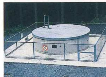
Drainage Well works (RC segment)
