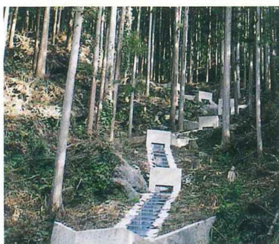
A water channel for leading groundwater to drainage.
