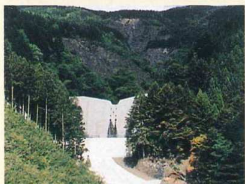
Kamekubosawa in Abe River drainage (Kuchisakamoto, Shizuoka City). The highest check dam in Shizuoka Prefecture, H: 26m, L: 81m (Heisei 1th (1989))
