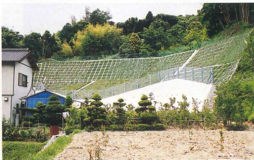
Finish walls and frames in Prevention works
