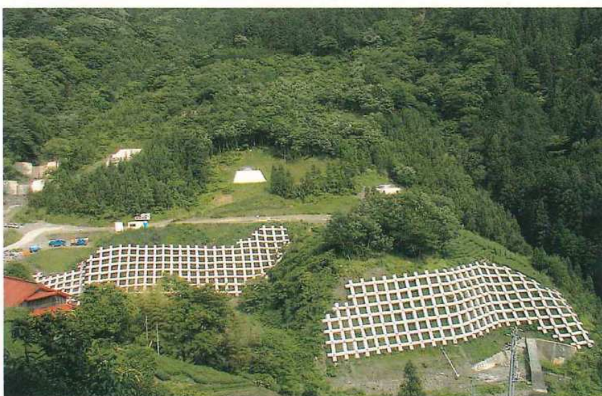
Landslide prevention works accomplished Slope frame and anchor works
