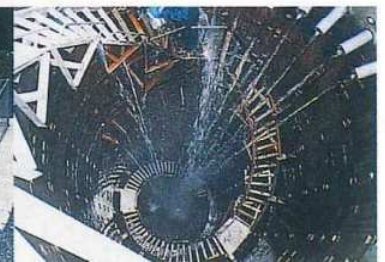
Draing groundwater from a catchment well.
