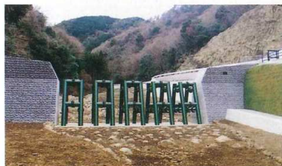
Umeki No.4 check dam with measures against debris flow driftwood (Izu city)
