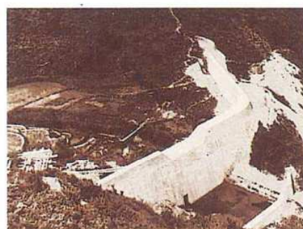
Sugegaya River in Hagima River drainage (Sugegaya, Sagara Town, Haibara County). Erosion control works in Showa 27th (1952). It was the biggest dam at that time in Shizuoka Prefecture and is still used as a reservoir dam.
