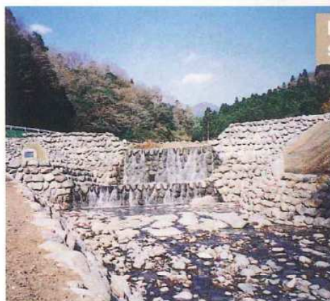
Check dam using local generating materials
