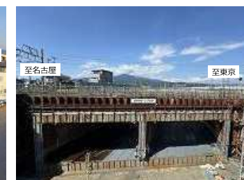
掘削完了R6.9
